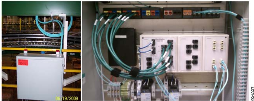
Figure 11 Sample Network Zone Fiber Optic Deployment
